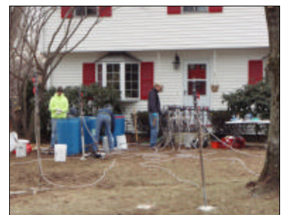
BEI scientists perform in-situ remediation on contaminated soil at a residential property
